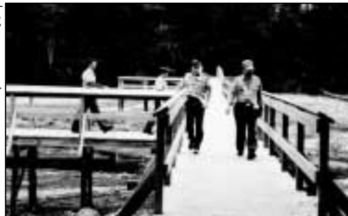
From left: Section SR 4 Section Chief Devlin Cooper, 2000 Lodge Chief Jeremy Stinson, 1999 Lodge Chief Kevin Right, and Lodge Adviser Ross Cooper walk along the new bridge constructed by the Echeconnee Lodge.
